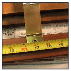
Step 3: If the decision to proceed is made, center the hinge on the back rail of the music desk. The hinge connected to the shorter of the two extension pieces goes here, with the bevel for the screws up. The furthest forward position is pictured, with the leading edge of the hinge in line with the edge of the back rail. This will provide the steepest slant possible for the music rack.
