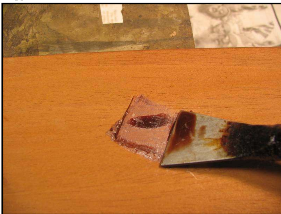
Photo 2: Slowly work the blade across the patch
