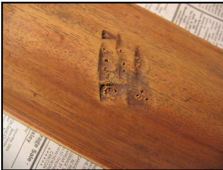
Photo 5: Badly damaged fallboard with anchor holes drilled
